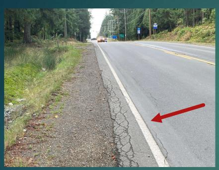
Shoulder is very narrow and degraded to point of being dangerous
